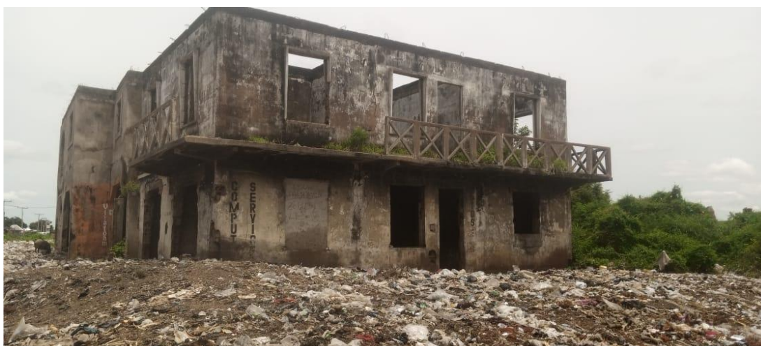
Figure 2. A razed house in Wukari. It shows a strong reminder of how the violence destroyed families, culture, and safety during the peak of the conflict.
