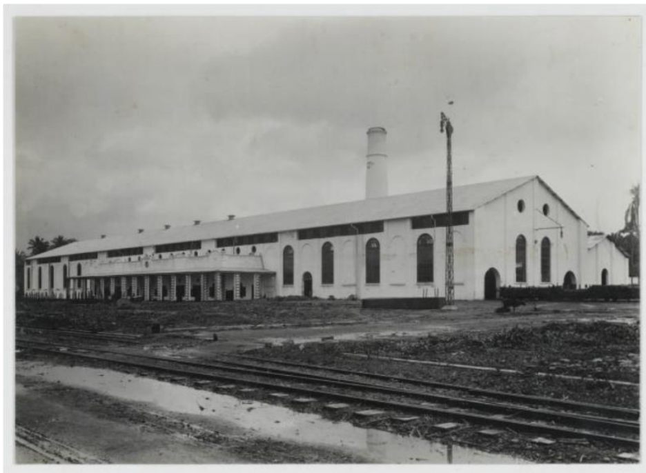
Figure 1. The Klampok Sugar Factory building seen from the exterior Source: [23]
